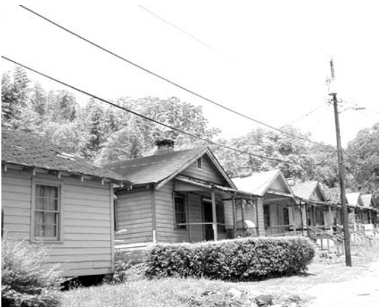
Figure 10.6 Traditional Southern ‘Shotgun’ Houses. Although some of these houses were too decayed to be rehabilitated, others could be saved. This modest housing type can usefully serve as a model for new affordable housing in the community.
